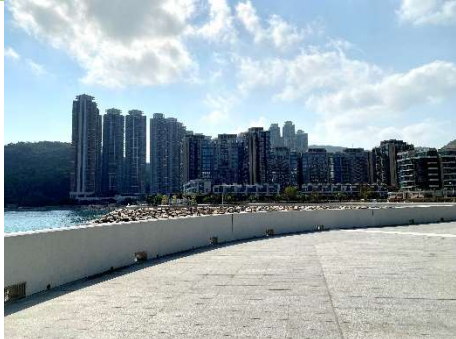
Wave wall to minimise overtopping wave.
